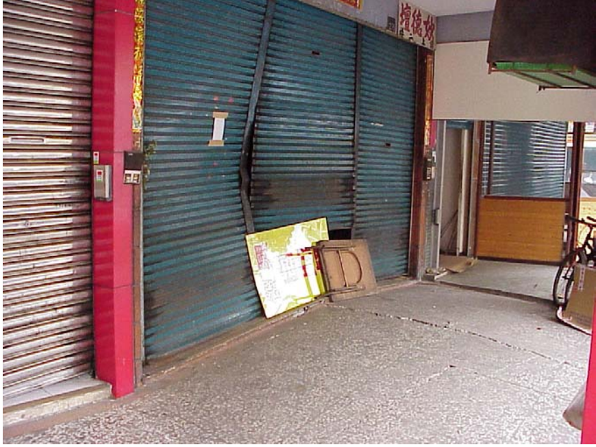
Fig. 2. Floating floor slab fractured by 25 cm settlement at walls/columns
