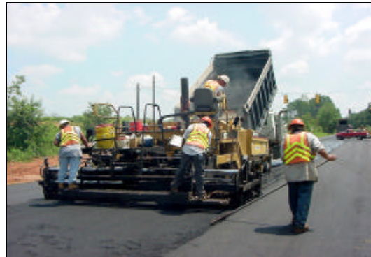
Asphalt pours from the dump truck into the paver and is laid at temperatures exceeding 300°F
