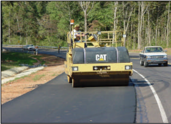
Figure 2: Compaction of the rubber modified HMA was similar to that of most HMA mixes
