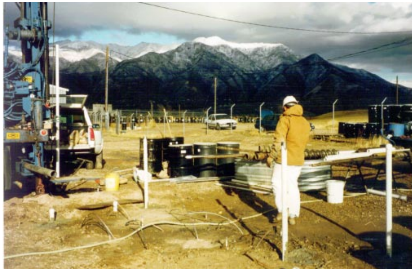
Installation of multi-level samplers and wells at the cosolvent injection site, Hill Air Force Base, Utah
